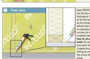
Apply ORCON joint adhesive, forming a continuous bead approx, 5 mm thick on the floor board and lay the membrane in the adhesive bed, leaving an expansion joint. Do not press the adhesive completely flat. Note for all adhesive bonds: The substrate onto which the adhesive is applied should be load bearing, dry, smooth and free of dust, silicon and
